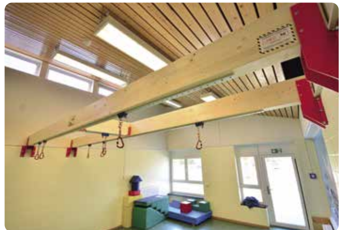
Ev. Kindergarten in Herne
